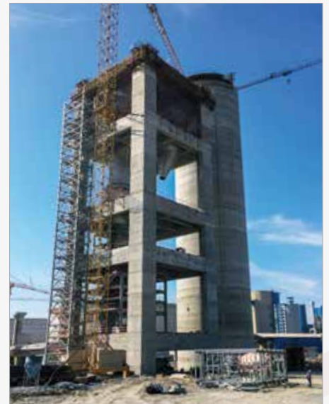
Concrete Pumping at 175 m Height
