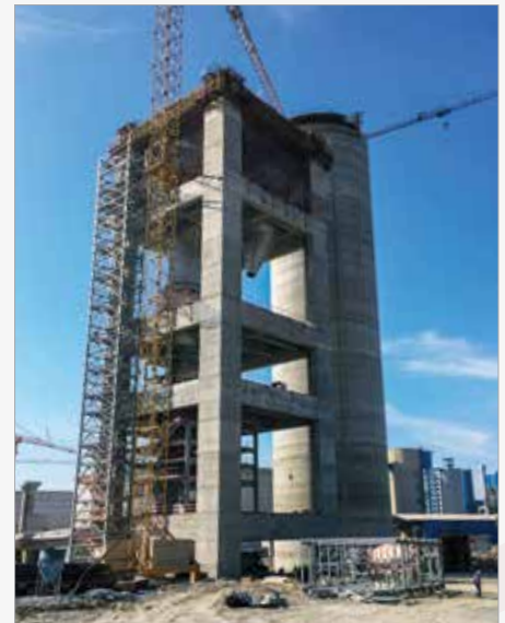
Concrete pumping at 175 m height
