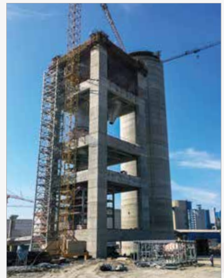
Concrete Pumping at 175 m Height
